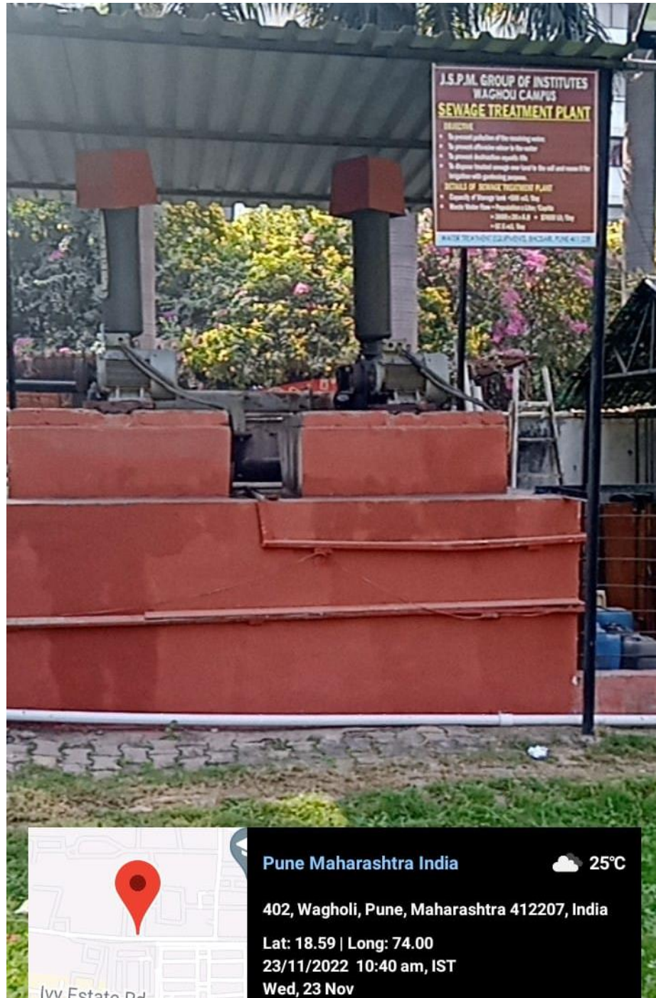
Fig. 7 Sewage Treatment Plant at ICOER
