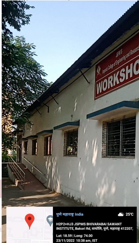
Fig 13 Ramp at central workshop of ICOER
