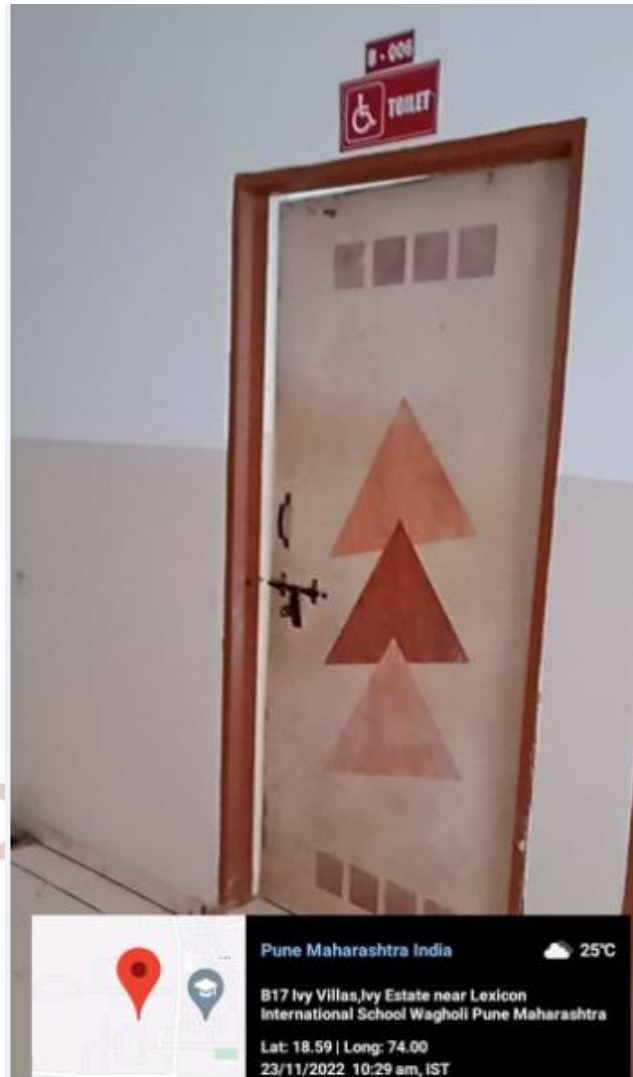
Fig. 14 Toilet for disabled of ICOER
